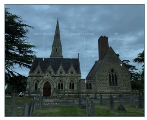
Figure 1. South elevation of the Old Chapels. Including the South Chapel, Transfer Corridor and Old Crematorium. Note cast iron hoppers and down pipes and steeply pitched roof of the Old Crematorium.
