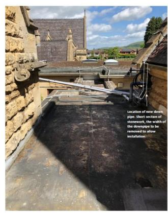
Figure 8. View north of the flat roof above the Transfer Corridor. New down pipe to be installed at this end of the Old Crematorium roof. Exact arrangement of new downpipe to fit around existing pipes.
