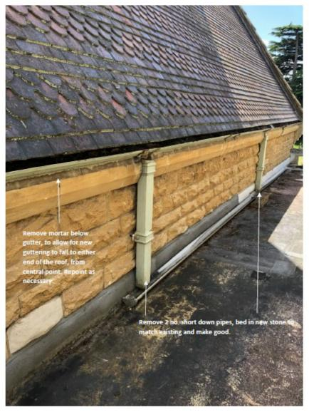
Figure 4. Close up of gutter and downpipes on Old Crematorium roof.
