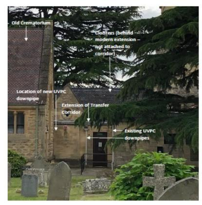
Figure 11. View of the east elevation of the modern extension of the Transfer Corridor. Note the existing UVPC hopper and downpipes.
