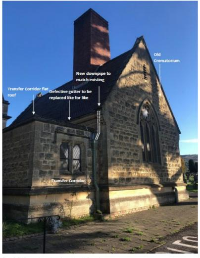
Figure 2. Old Crematorium and transfer corridor with flat roof.
