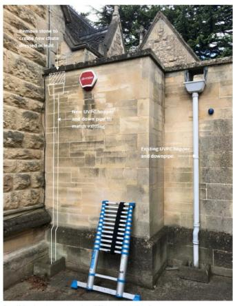
Figure 10. New down pipe to match the existing UVPC down pipe in the right of image.
