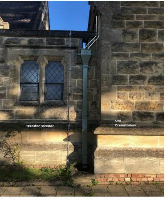
Figure 7. Close up of the existing down pipe on the front elevation of the transfer corridor. The new down pipe will link the gutter to this downpipe.
