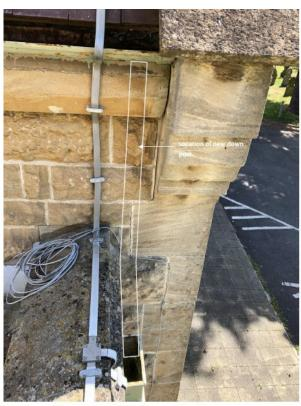
Figure 6. Close up of the location of the new pipe, linking the gutter to the hopper below.
